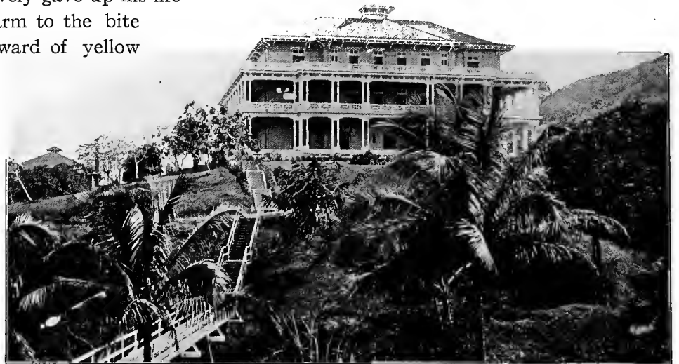
ADMINISTRATION BUILDING, HOUSING THE SANITARY DEPARTMENT
